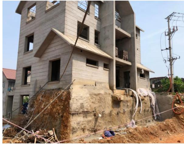
Figure 10. Site visual assessment of stability of the building after excavated.
