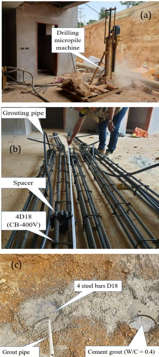
Figure 3. Design and construction of micropiles at the study building.
